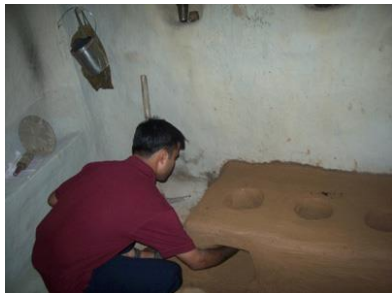
Installation of smokeless chulahs by a lodge associate with the help of a villager.
