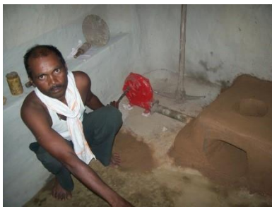
Installation of smokeless chulahs by a lodge associate with the help of a villager.
