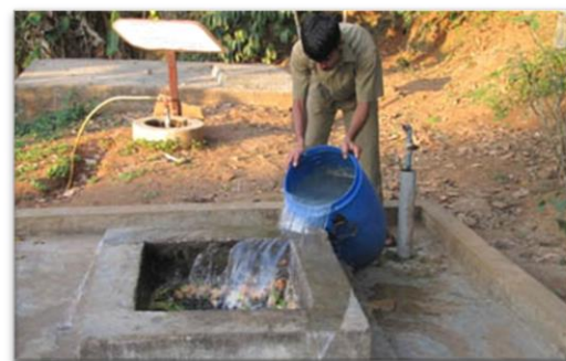
Biogas unit using food waste to power cooking.
