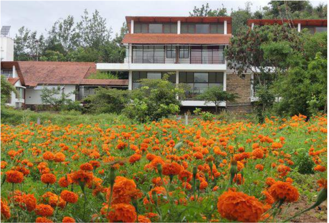
Large windows, sliding doors and wide eaves maximise the use of natural light and ventilation.
