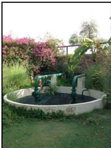
300 feet well for rainwater harvesting.
