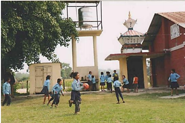
Water tank and second school building provided at the local school.
