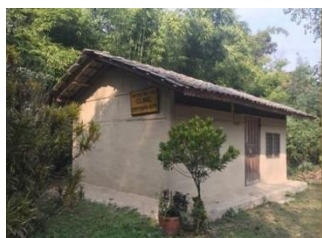
On-site village health clinic.
