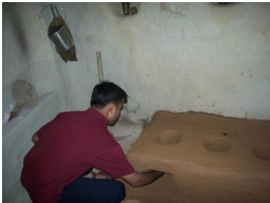
Installation of smokeless chulhas by a lodge associate with the help of a villager.
