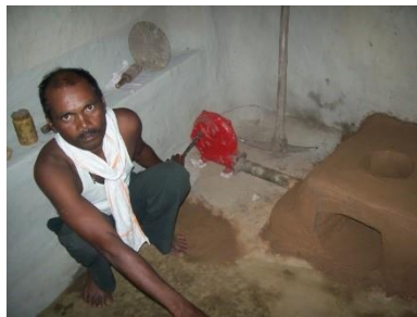
Installation of smokeless chulhas by a lodge associate with the help of a villager.
