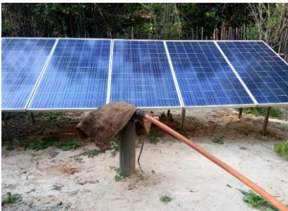
King's Lodge, Bandhavgarh uses a solar water pumping plant for ground water.
