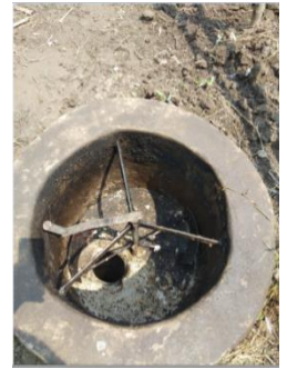
Biogas unit converting biodegradable waste into fuel for cooking.
