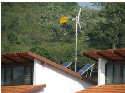
Micro wind and solar power hybrid generator.
