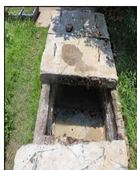
Grease trap skimming of oil and fat from the kitchen.
