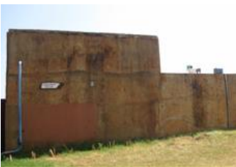
Sewage treatment plant.
