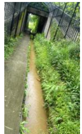
Pathway created on the lodge premises to enable villagers to access a free-flowing water channel.
