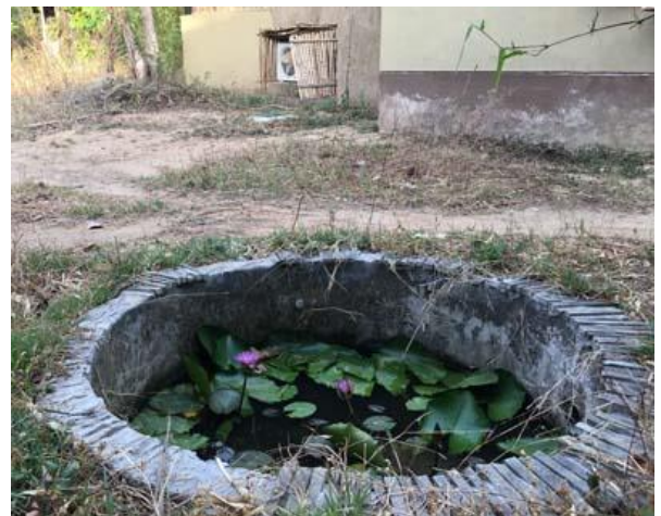
Grey water from cottages passes through filtration pits to lily ponds.
