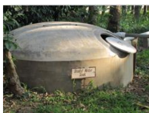
Treated water is recycled for irrigation saving water. Sludge is converted to organic manure for use on neighbouring farms.
