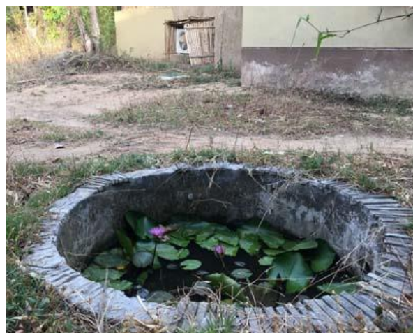
Grey water from cottages passes through filtration pits to lily ponds.
